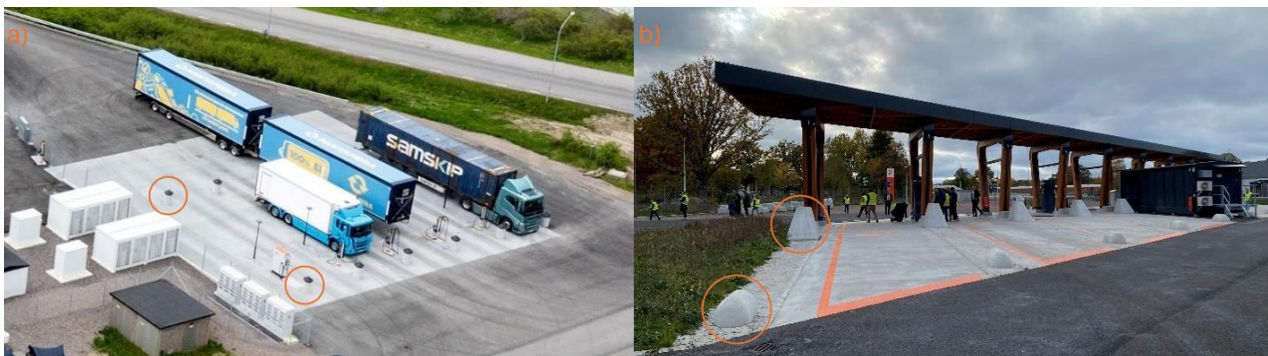
Figure 14 a) Charging station Alfredsson Energy, Sweden, where it is clear that they have used another pavement where the chargers are to better adapt to the static force. The orange circles mark their anti-collision solutions. Image from Alfredsson Energy. b) Milence station at Ödeshög, Sweden, the surface at the charging bays is different from the surrounding surfaces. The orange circles mark their anti-collision solutions. Image from Lindholmen Science Park.
