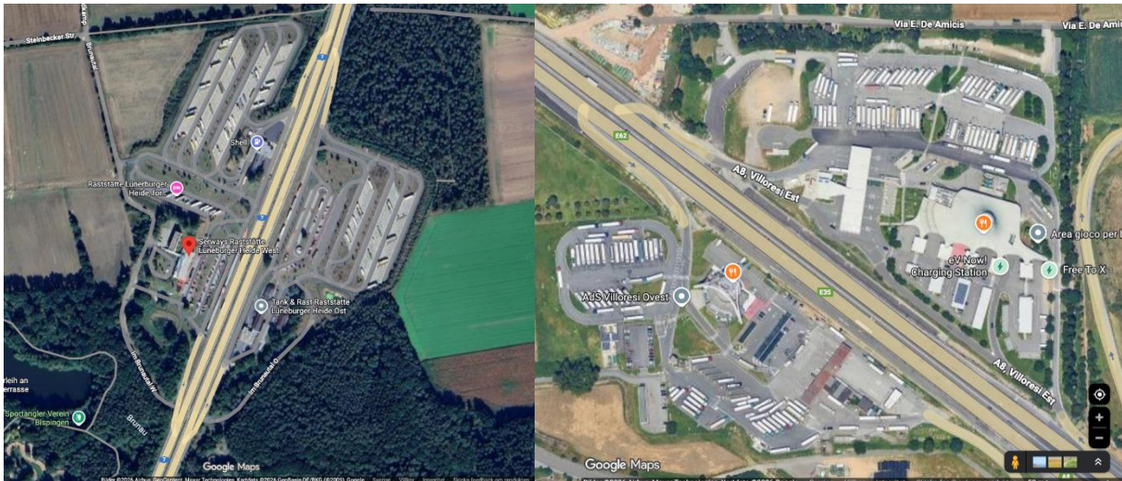
Figure 10 Examples of larger rest areas in direct contact with the motorway. Raststätte Lüneburger Heide, Germany (Left) and Autogrill Villorresi Est, Italy (Right). Images from Google Maps,
