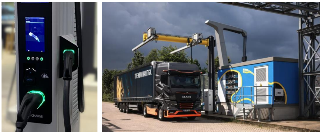
Figure 19 Examples of combined CCS and MCS hardware. A Siemens charging point with both MCS and CCS (left) and Shell Amsterdam ETCA charging site with a combined over-head CCS and MCS charger which shares power electronics with MCS charger for ships (right). Images from Lindholmen Science Park and Shell.
