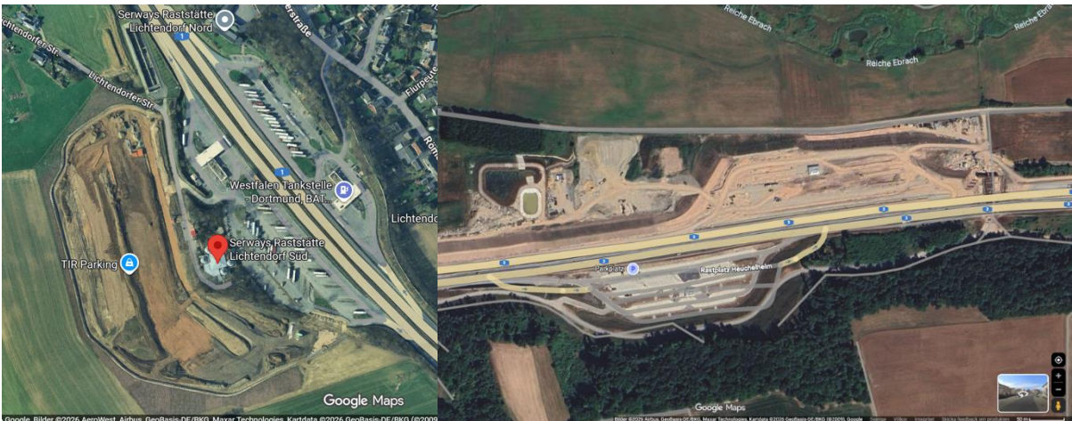
Figure 6 Example of expanding rest area a) Lichtendorf Süd, in Nord Rhein Westfalen, Germany b) Rastplatz Heuchelheim, Germany. Images from Google Maps.
