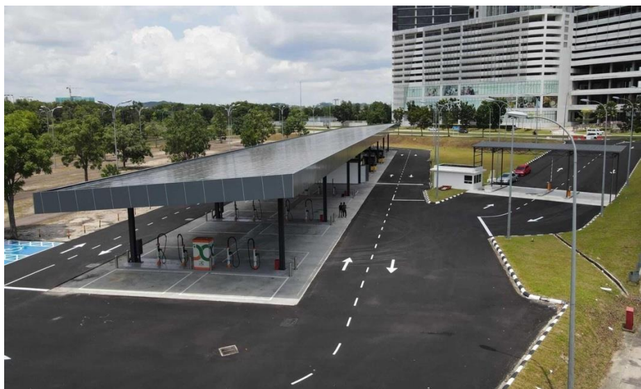
Figure 12 DC Handal Mall of Medini EV charging hub, Malaysia, is a site adapted for both LDVs and HDVs such as trucks and buses. One HDV can fit in two charging bays for LDVs. Image from Kempower.
